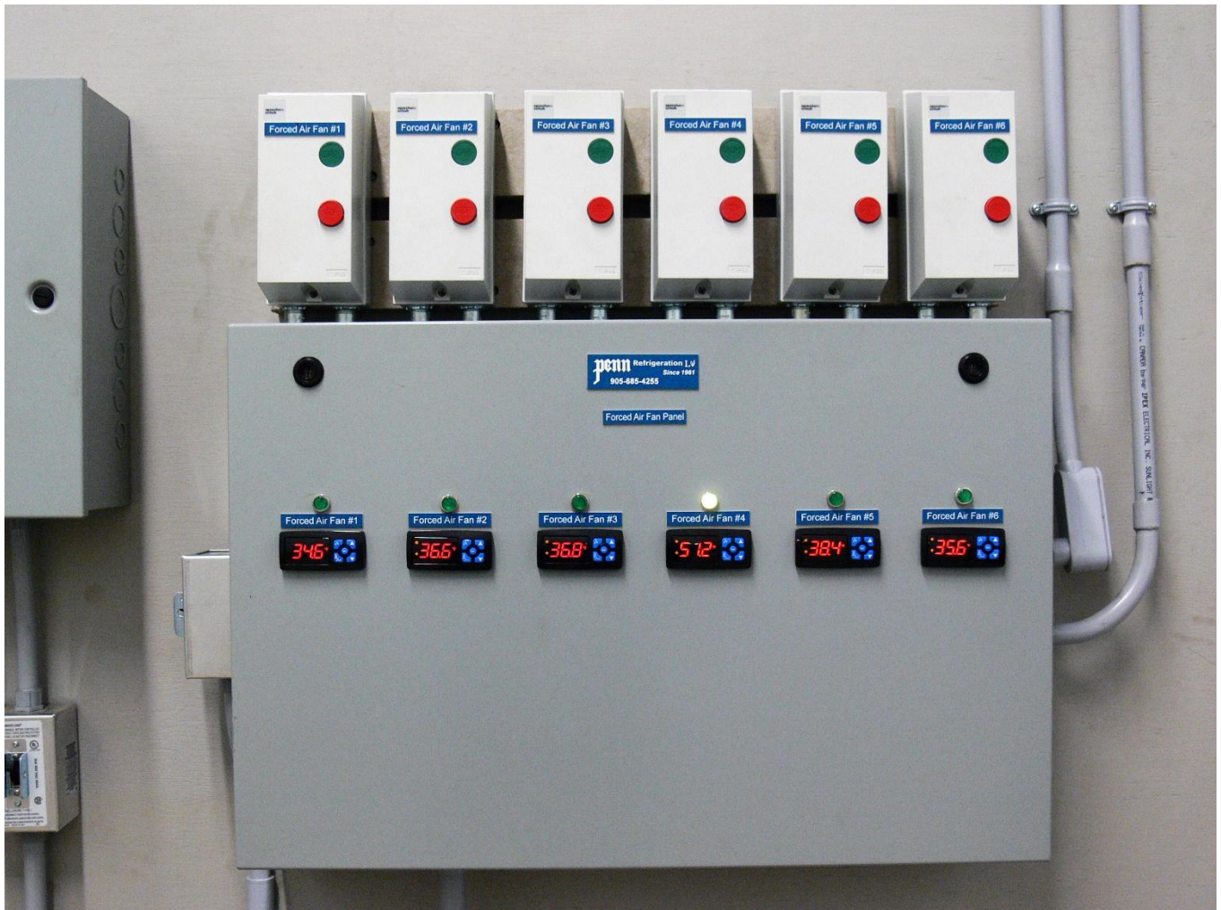
Figure 6. Sensors monitor “warm” air temperatures (°F) exiting the column of bins in the serpentine horizontal/vertical airflow system in Figure 4. At the time of this picture, cold air entering Forced Air Fan #4 was 35.6°F (2°C) and the internal temperatures of three individual, equally sized pears being monitored were 59°F (15°C), 67°F (19°C) and 68°F (20°C) along the cooling path, averaging 64.4°F (18°C). Fruit started at about 71.6°F (22°C), so the temperature at Fan #4 (51.2°F; 10.7°C) is about halfway between the cold air entering at 35.6°F (2°C) and the average internal temperature of cooling fruit at 64.4°F (18°C). With experience, one can make good predictions about internal fruit temperatures at any time within the bins. (Photo by Hugh W. Fraser, OMAFRA)
