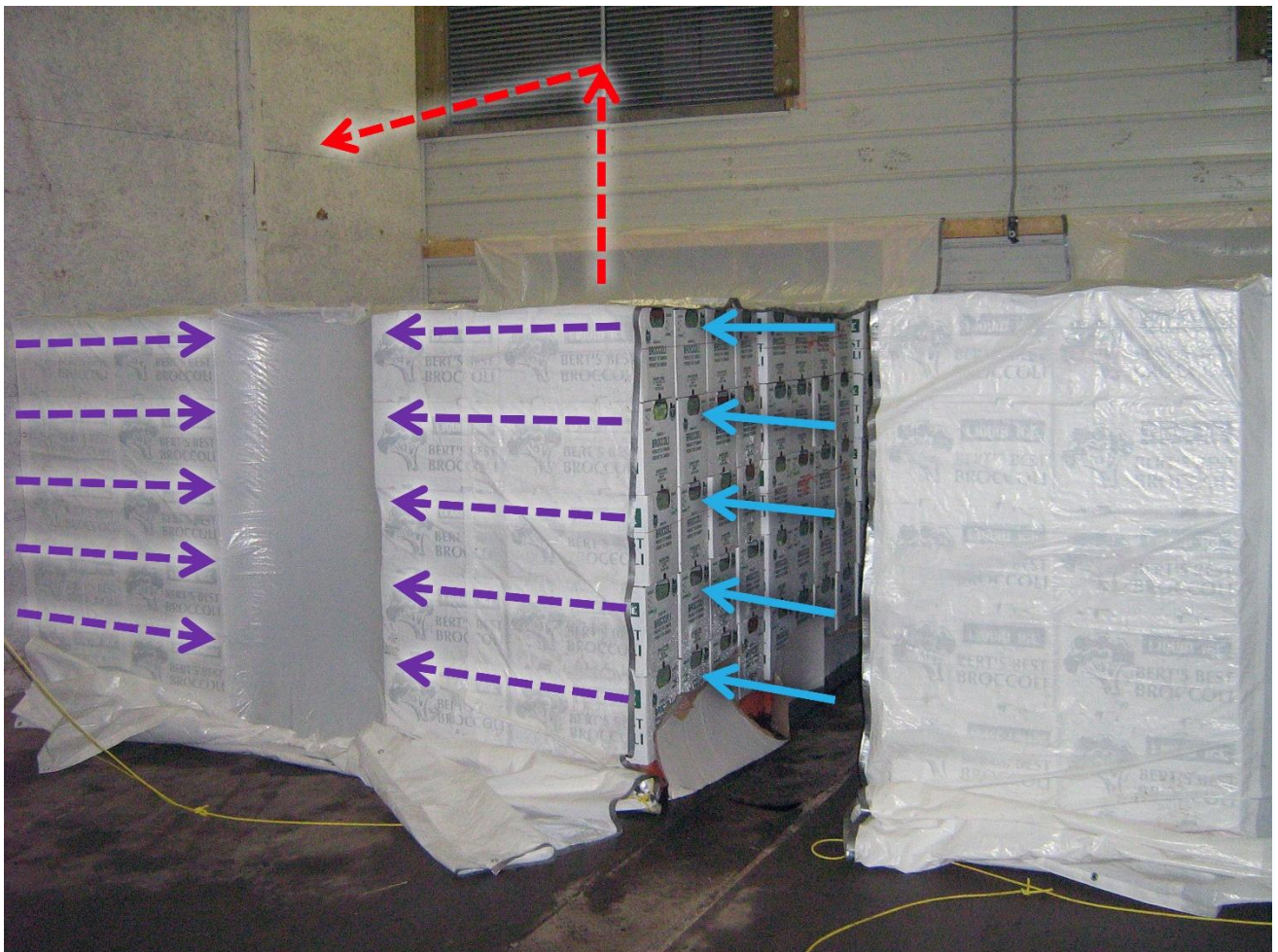
Figure 2. This tunnel horizontal airflow system has high-capacity fans inside a plenum (located behind the pallets) that pull refrigerated air (blue arrows) from the room horizontally through produce boxes. Warmed air (purple then red arrows) then travels through a “tunnel” created between the pallets and into the plenum, where it is directed back into the storage room (red arrows) towards the evaporator coils to be re-cooled. Pallets are cooled in pairs. Plastic sheeting sucks tightly against the boxes and tunnel. Sheetting is swung into place with cords attached to the ceiling.
